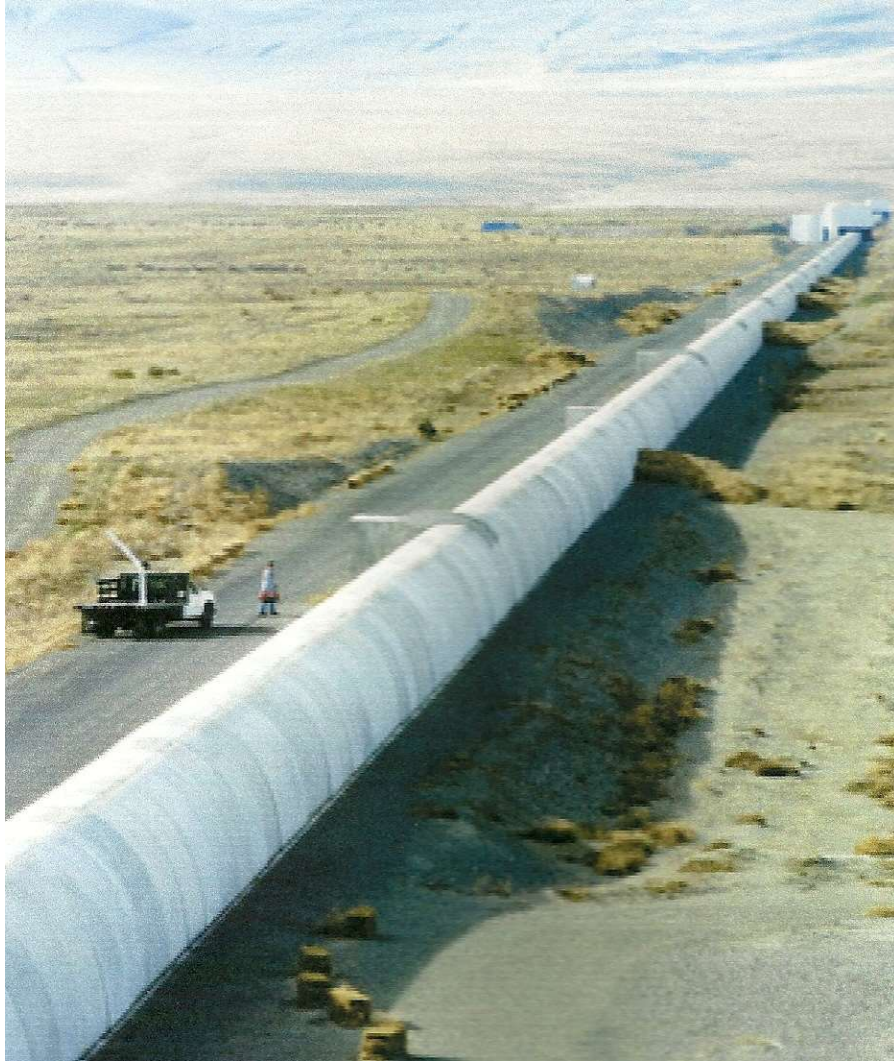
Four-kilometer long LIGO vacuum tunnel or Interferometer “Leg” by NASA.
